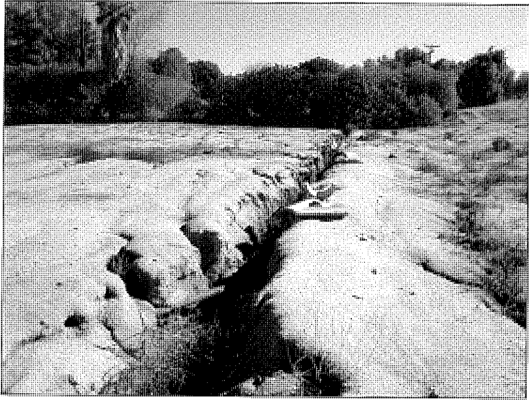
Typical deep surface erosion at isolated locations.
