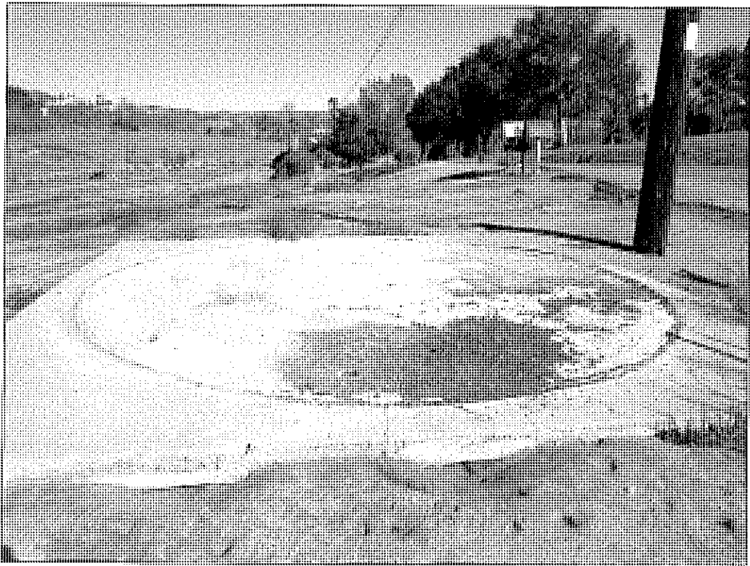
Concrete slab with remnant steel ring reportedly the location of a storage tank used to contain Oil. Dimensions 8' h x 12' diameter.
